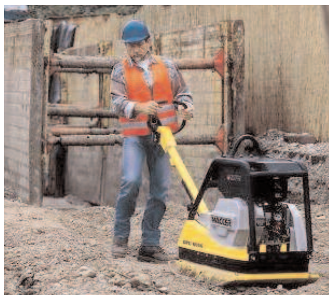
Figure 1 A compaction machine in use
