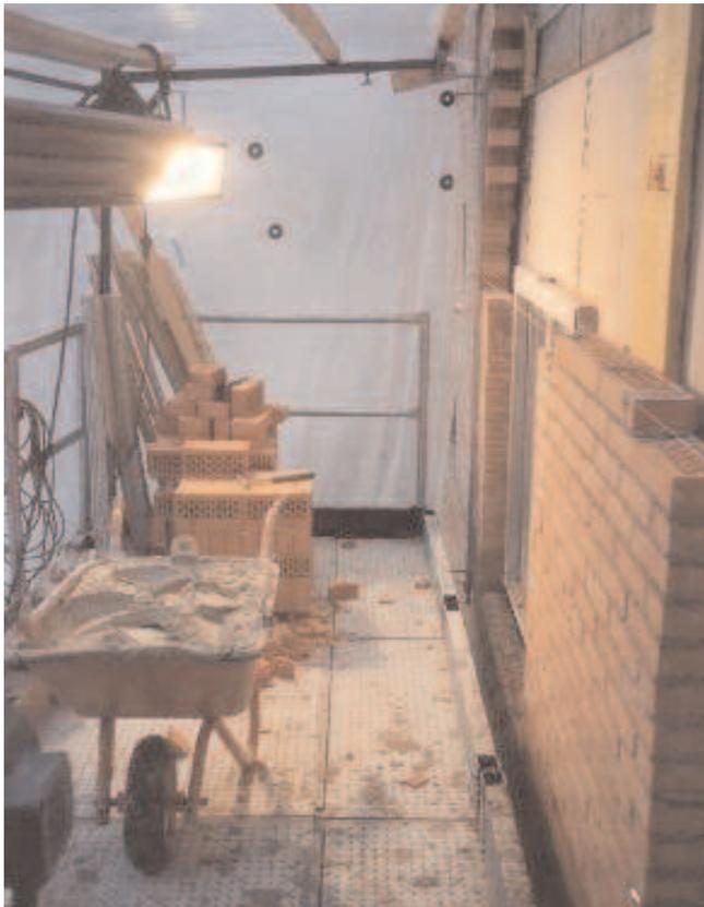
Figure 5 Lighting can be provided and the platform can be enclosed by netting to protect the workers
