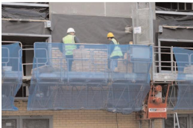
Figure 3 The working platform can be set so that the tradesmen can work at a comfortable height without excessive bending and stretching.
