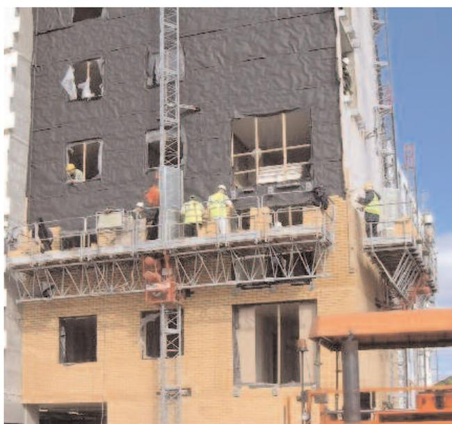
Figure 1 Mast climber being used for brickwork
