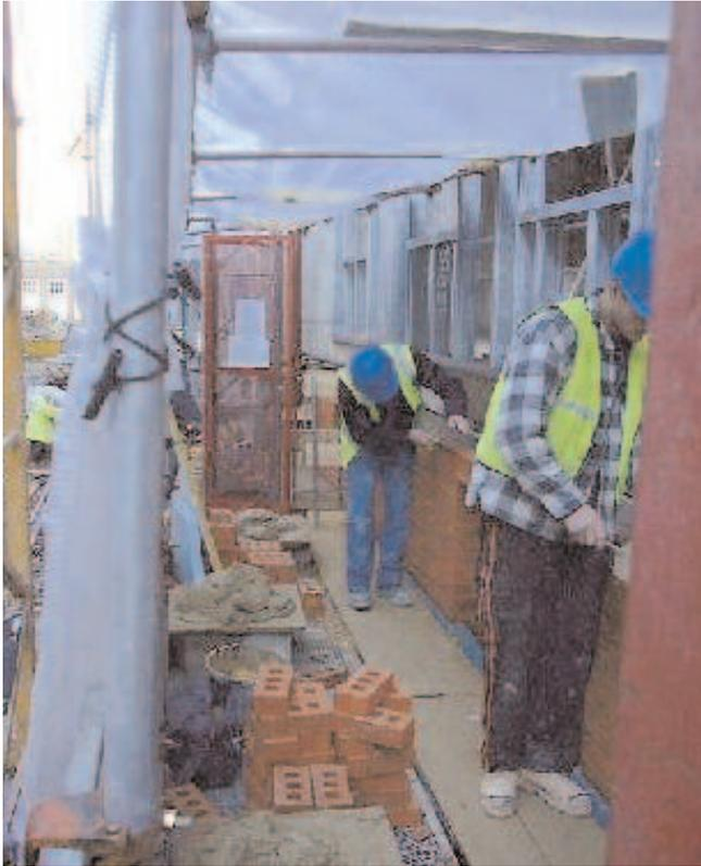
Figure 4 Bricklayers working from a mast climber. It allows them to work at about waist height and adopt a good posture
