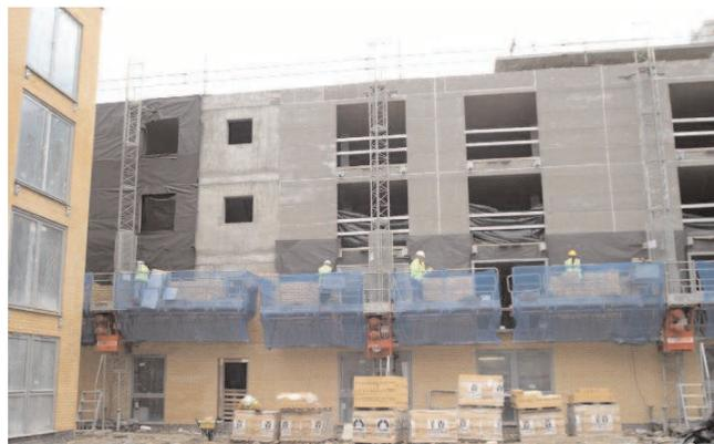
Figure 2 A series of mast climbers being used for brickwork
