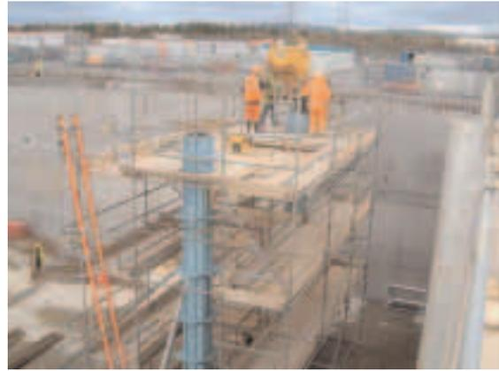
Figure 2 Improved formwork design following review
