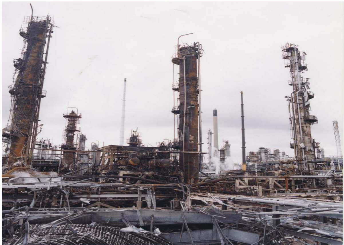
Figure 3 – Damage to the SGP after the explosion (W413 column to the right)
