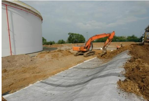
Installing a bund liner as part of secondary containment improvements
