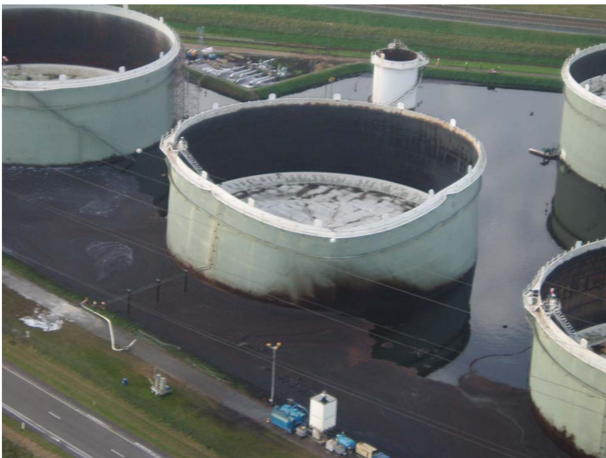
Figure 2: Picture of the situation in the bund the morning after the major accident
