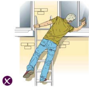
Figure 6 incorrect - oversaching and failing to maintain three points of contact
