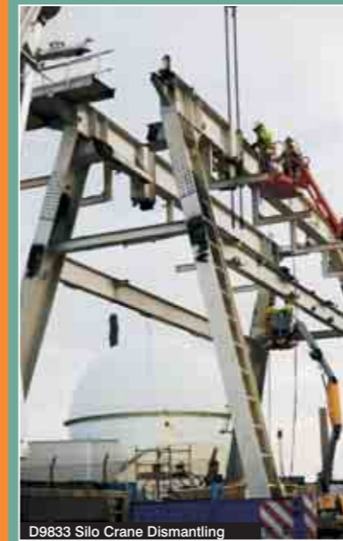
D9833 Silo Crane Dismantling
