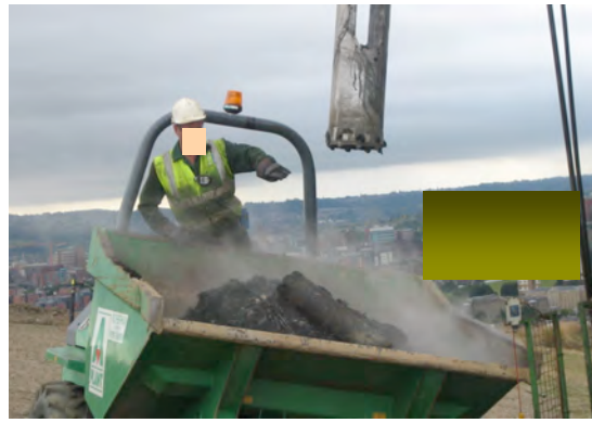
Figure 2 Emptying the auger.
