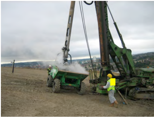
Figure 1 Emptying the auger.
