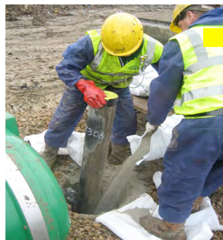
Figure 6 Capping the hole
