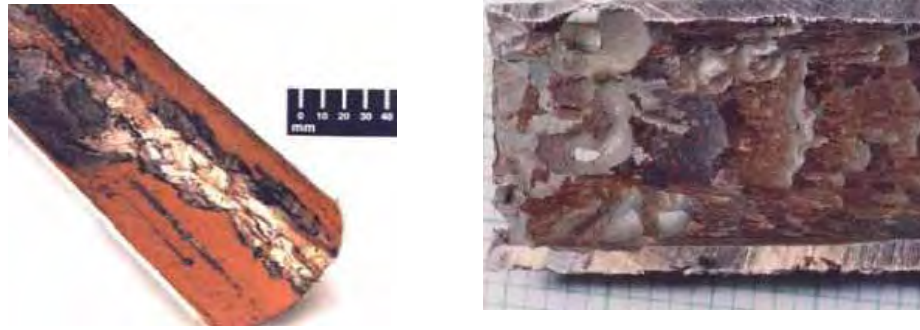
Figure 2: Examples of Erosion Corrosion
