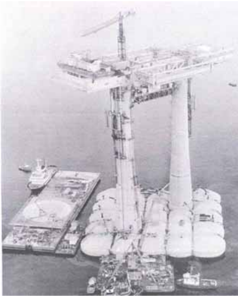
Concrete platform during construction
