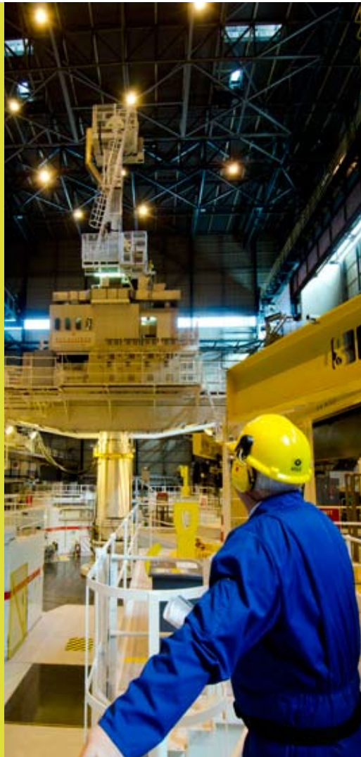
ONR inspector at Heysham 1 Reactor 2, looking along the common pile cap towards Reactor 1
