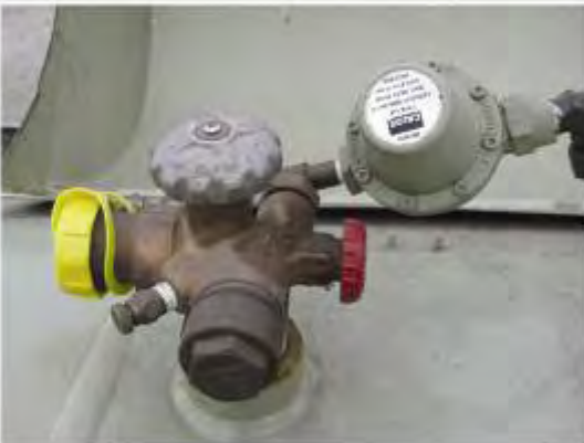
Multi-Valve unit With LPG fill connection, vapour off-take valve, maximum fill bleed valve + 1st stage regulator
