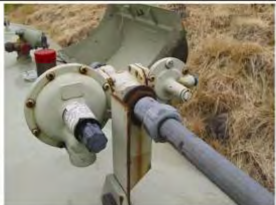
Combined 2nd stage regulator, UPSO & OPSO
