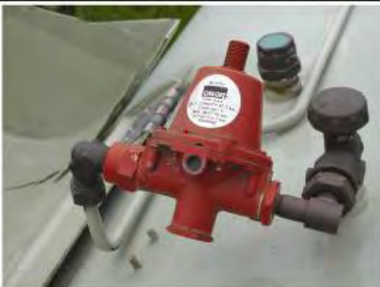
Multi-Valve unit With LPG fill connection, vapour off-take valve, maximum fill bleed valve + 1st stage regulator
