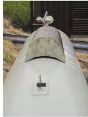
Lockable cover For the protection of combined multi-valve unit
