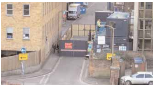
Figure 1 Road closure - good planning creates the conditions for effective worker engagement
