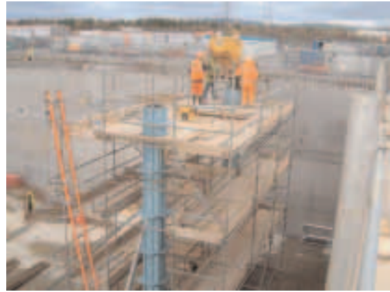
Figure 2 Improved formwork design following review
