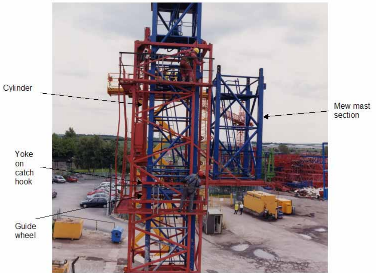
Figure 5 – Demonstration of climb at Castleford – prior to separation of mast head
