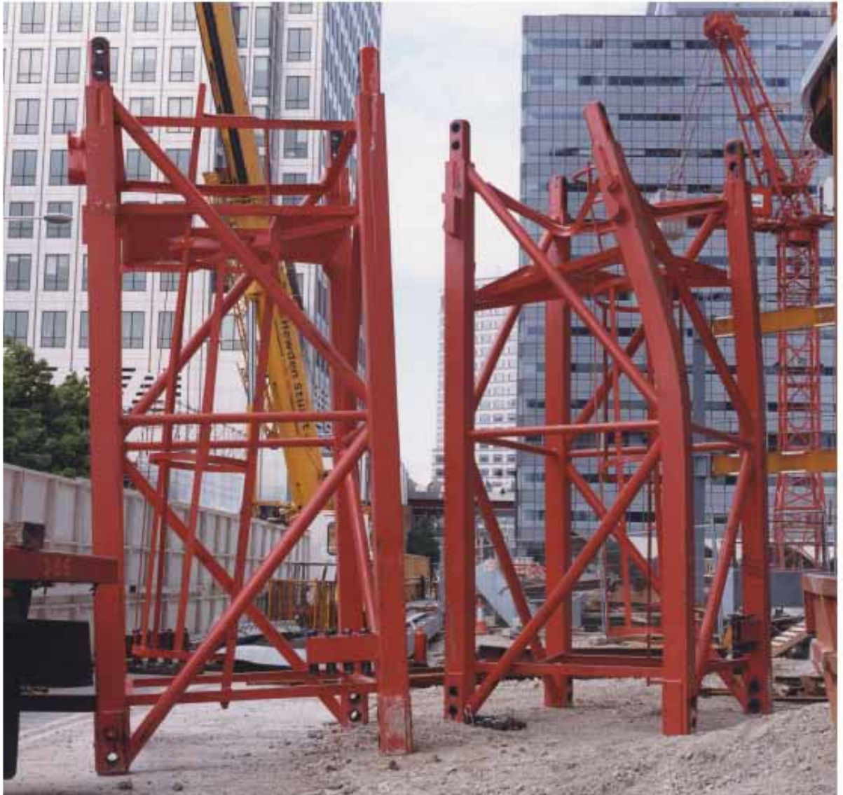
Figure 15 Two top mast sections of TC3 after recovery showing the pattern of damage
