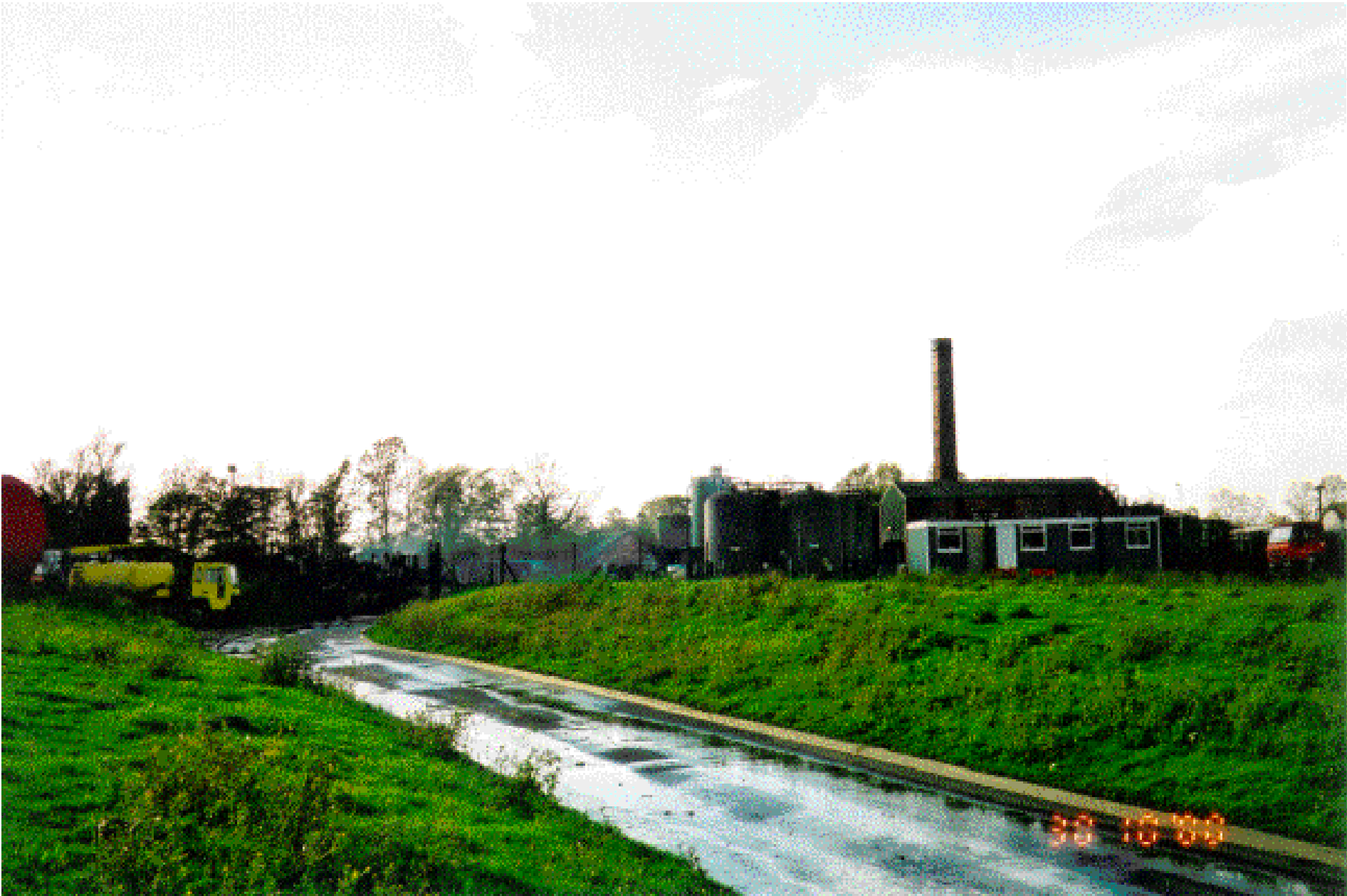
Photograph 1: Approach to site.
