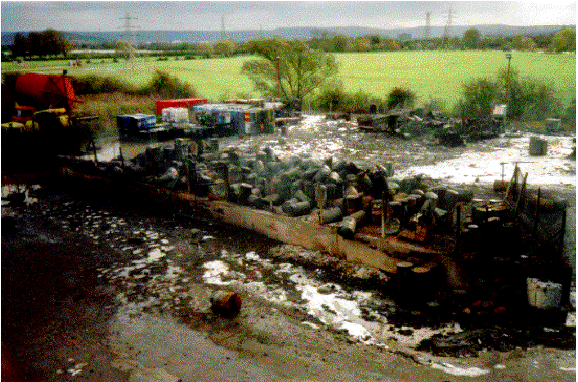
Photograph 2: Compound 3 after the fire.
