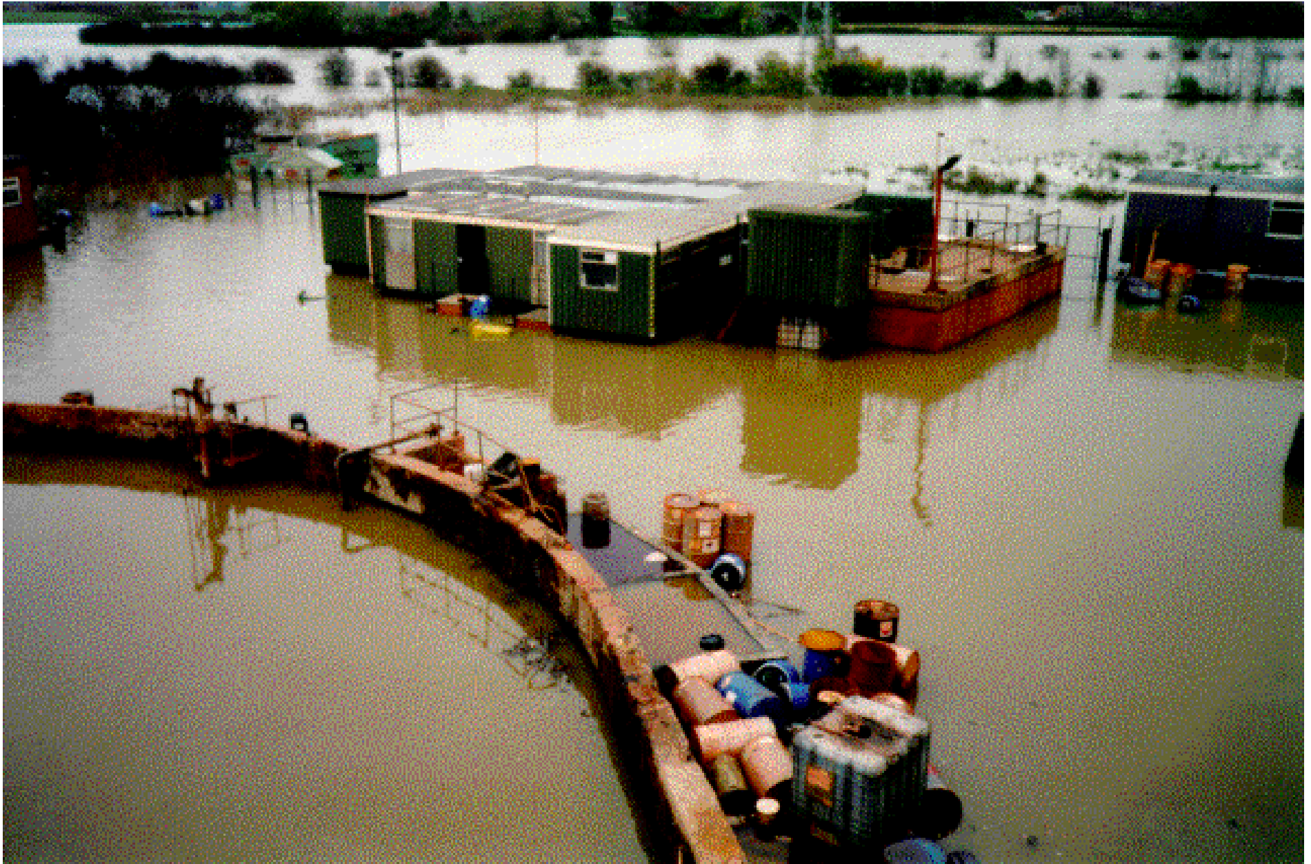
Photograph 8: View of part of large well and site offices during flooding.
